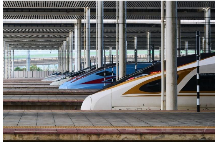
Picture 5: Different generations of High-Speed Trains in Guiyang
